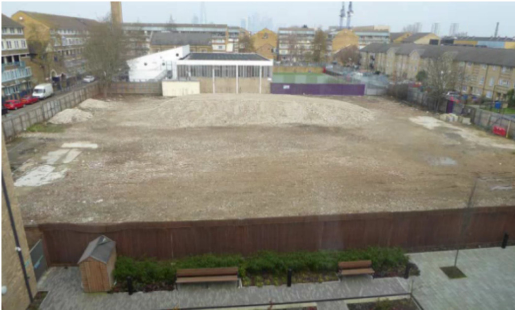
Figure 5: Photograph of the cleared TS2 site taken from the rear of TS1
